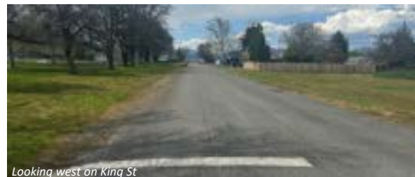
Looking west on King St
