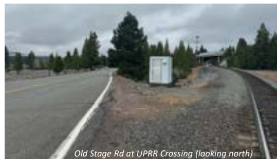
Old Stage Rd at UPRR Crossing (looking north)
