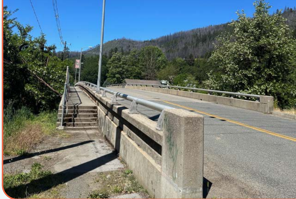
↑ 2nd Ave Bridge looking west
