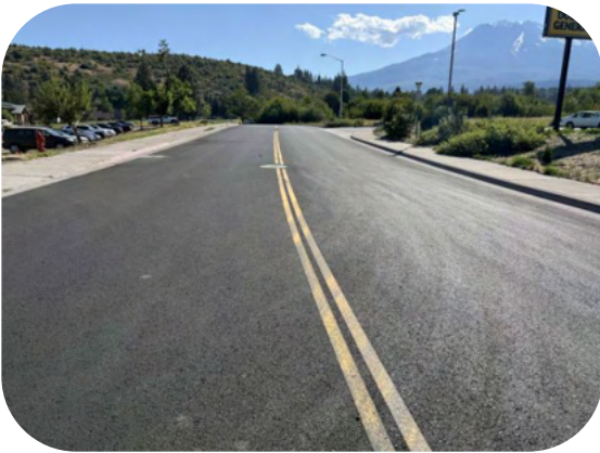
Boles & Mill Street STIP Project
